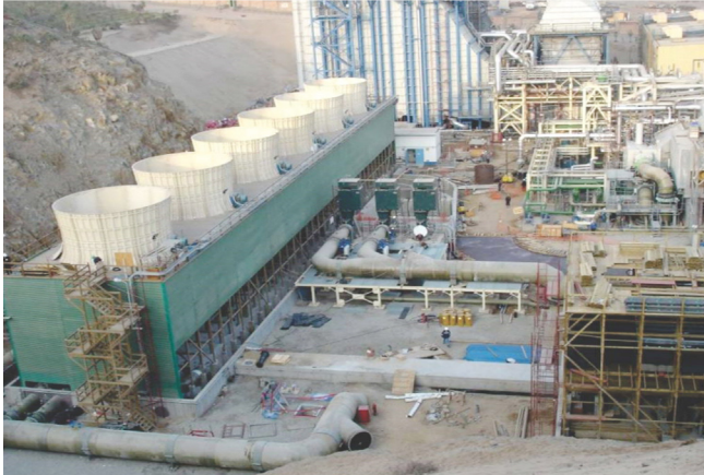
Figure 1: GRP Pipes Discharge
