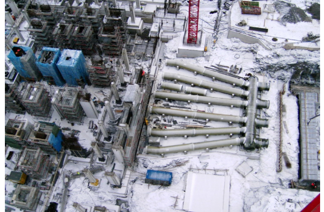
Figure 2: GRP Pipes Suction
