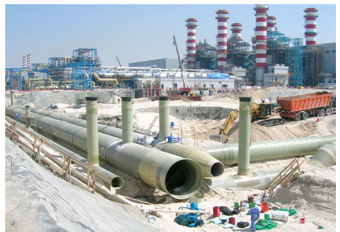
Figure 3: GRP Pipes Construction Site.
